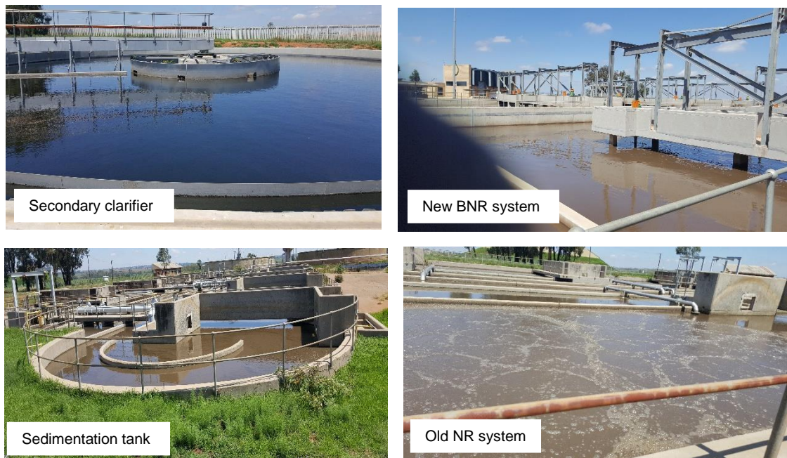
Figure 8: Section of Westonaria WWT plant
