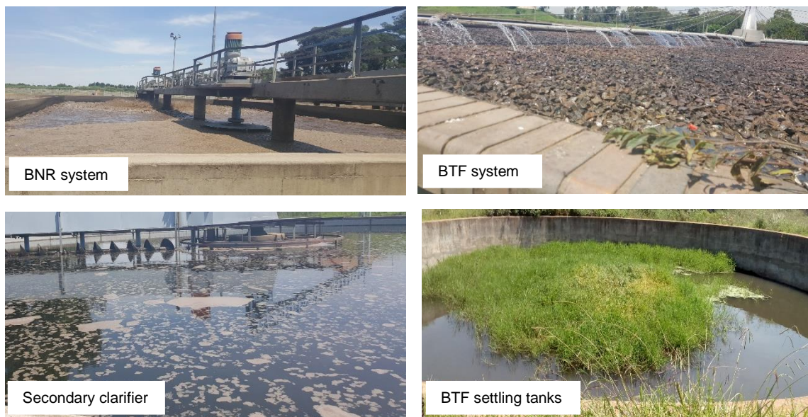
Figure 3: Section of Rietspruit WWT plant
