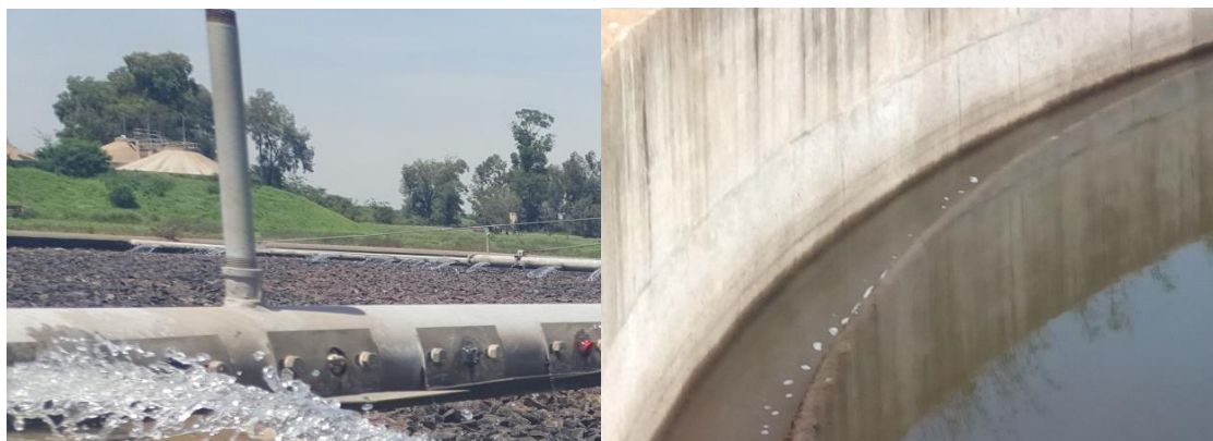
Figure 14; Biofilter system with turbid effluent discharged from secondary settling tank.
