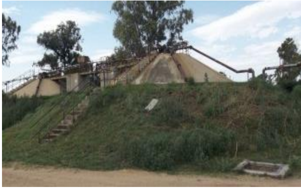
Figure 9 Anaerobic digesters, Plant XFSA
