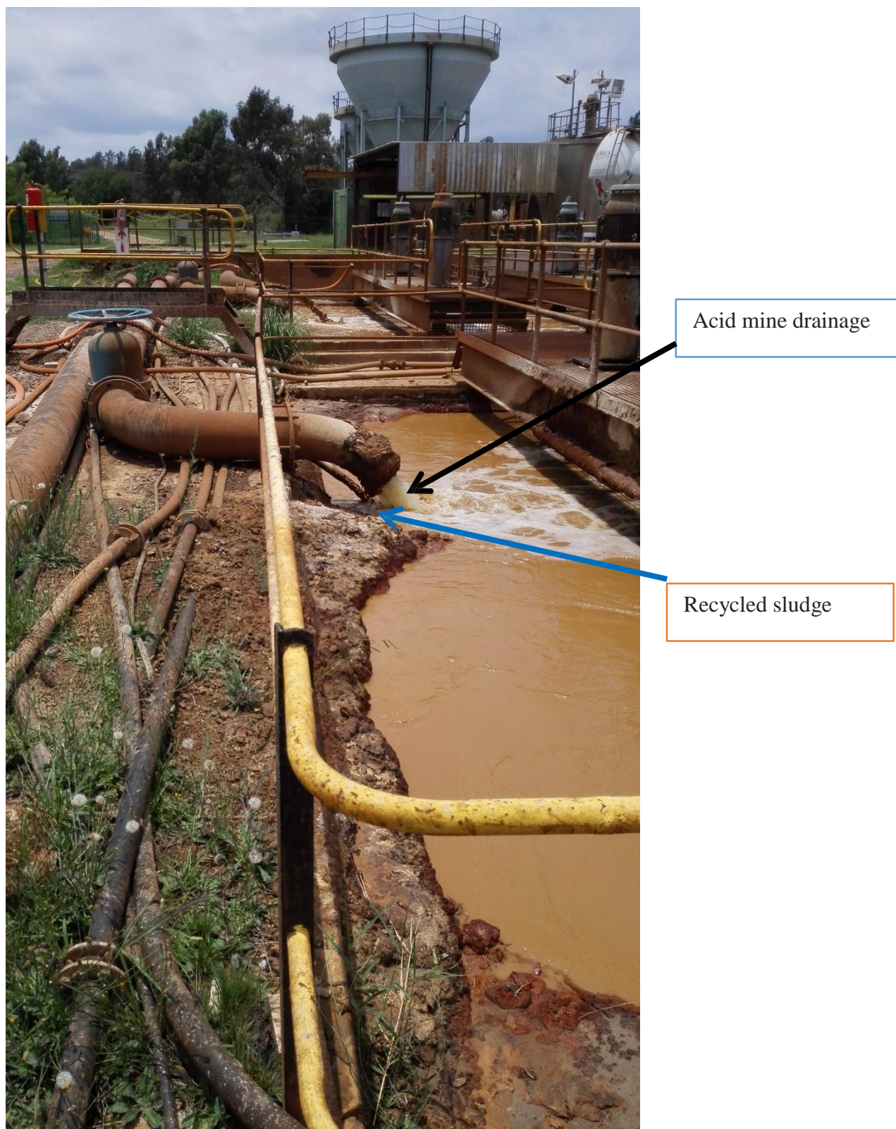
Figure 15: Acid neutralization plant, mixing tank.
