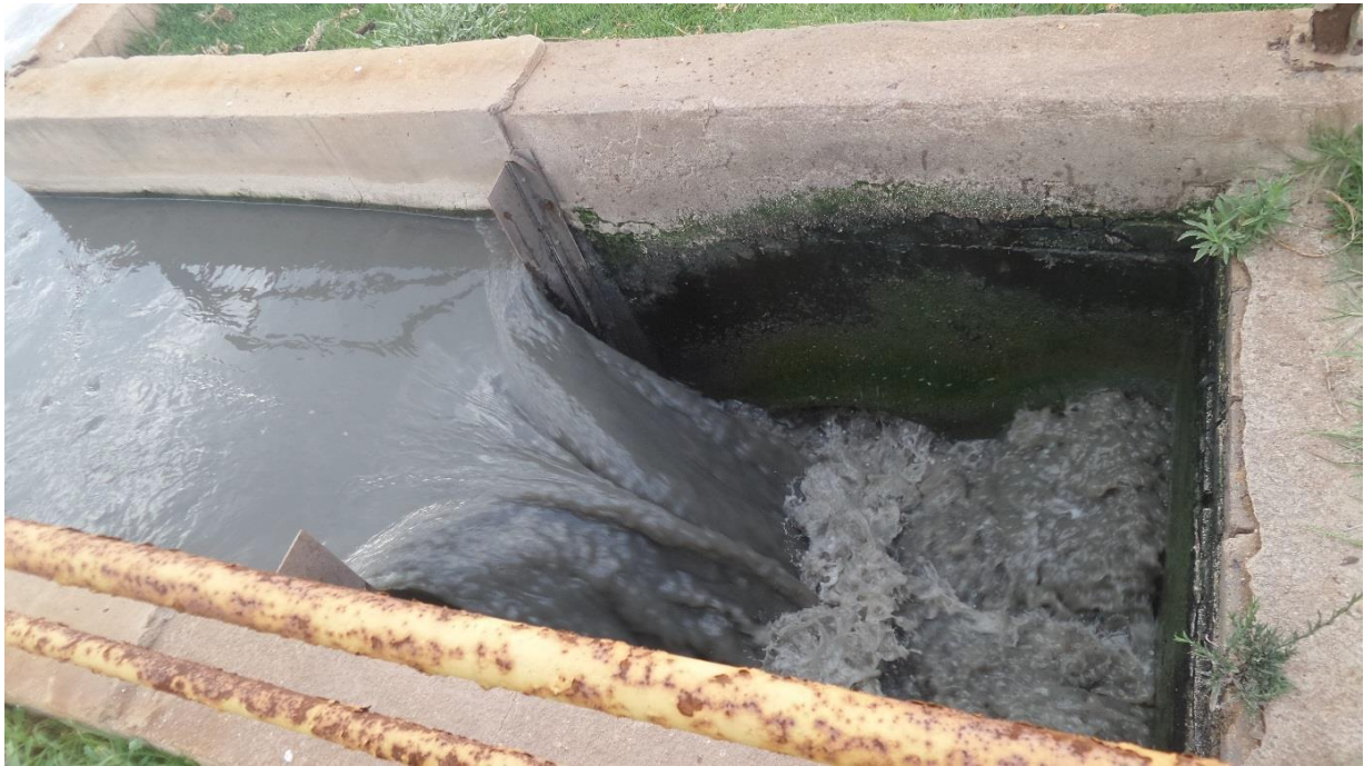
Figure 12 Effluent from an underperforming treatment plant (Plant XAMP)
