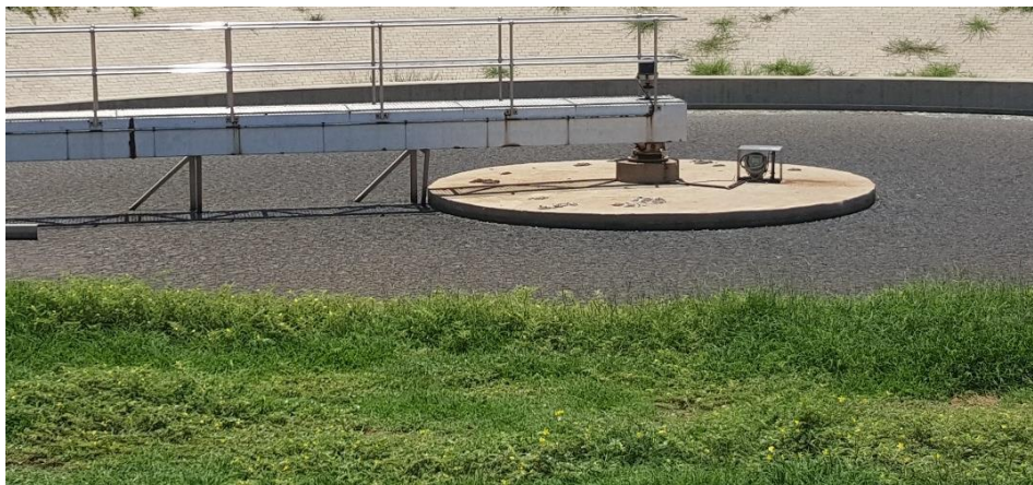
Figure 3 Flocculation unit (pond)
