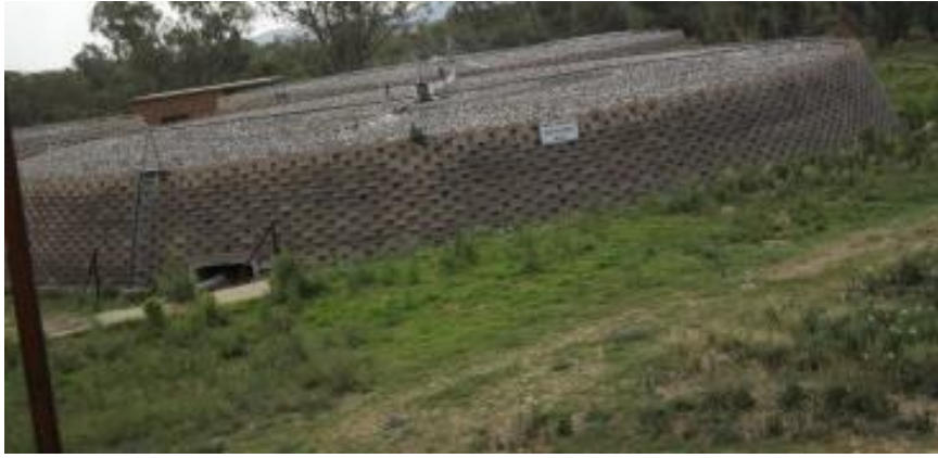
Figure 6 Biofilter unit at XFSA
