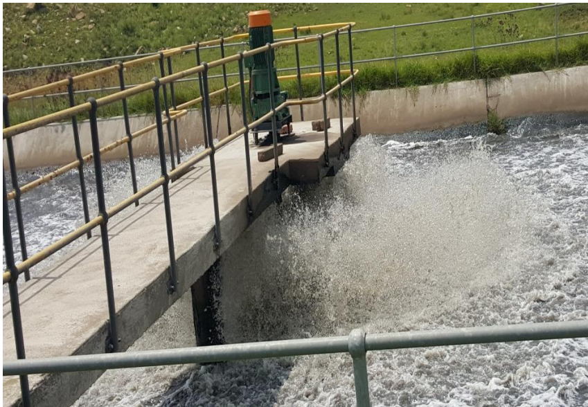
Figure 7 Aeration process, Plant XFSA
